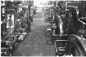
Steam Turbine (1890's)
